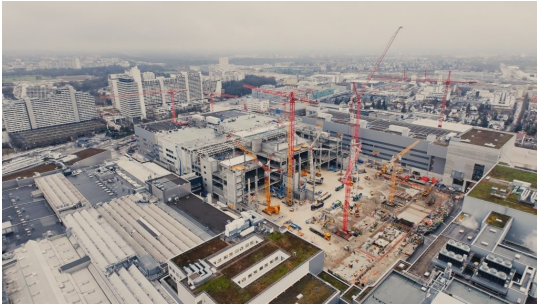
© BMW Group New assembly site in December 2024, BMW Group Plant Munich (02/2025).
